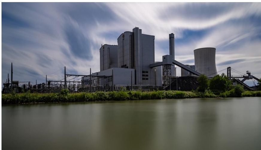
Abbildung 7.16, Kohlekraftwerk von: https://www.tu-darmstadt.de/clean-circles/transfer_outreach_cc/circular_economy_cc/index.de.jsp
