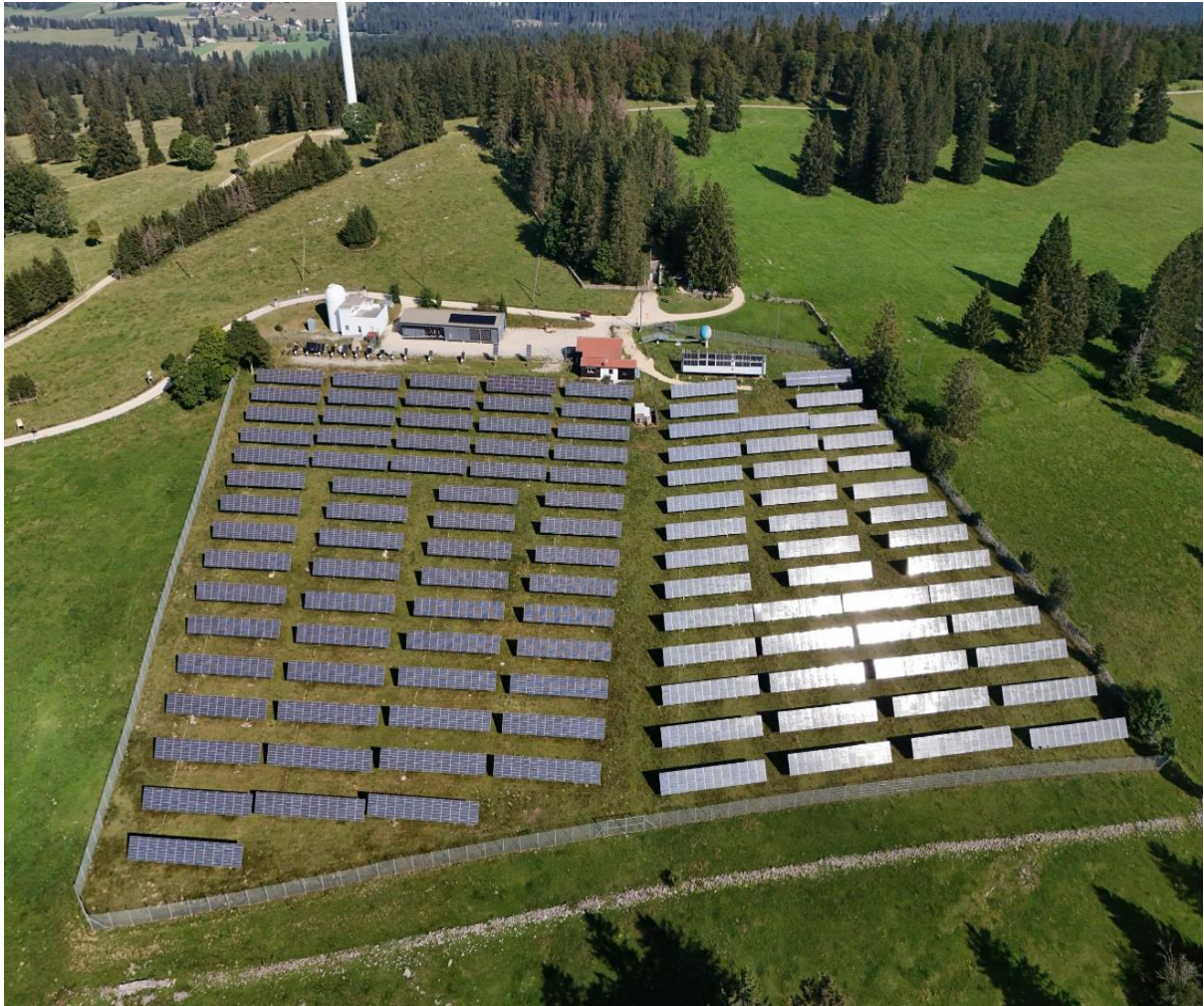
Abbildung 19 Solarpark Mont Soleil; Quelle: https://bkwfmbenergie.sharepoint.com/sites/T_BKWP_AM_PV_Switzerland/
