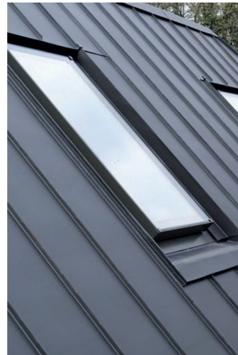
DACHFENSTER IN METALLDACH
